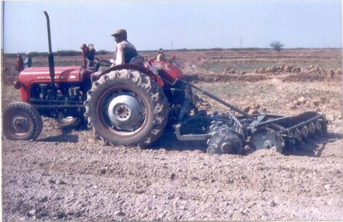
FIG 3. SOIL – FLYASH MIXING WITH A DISC HARROW
