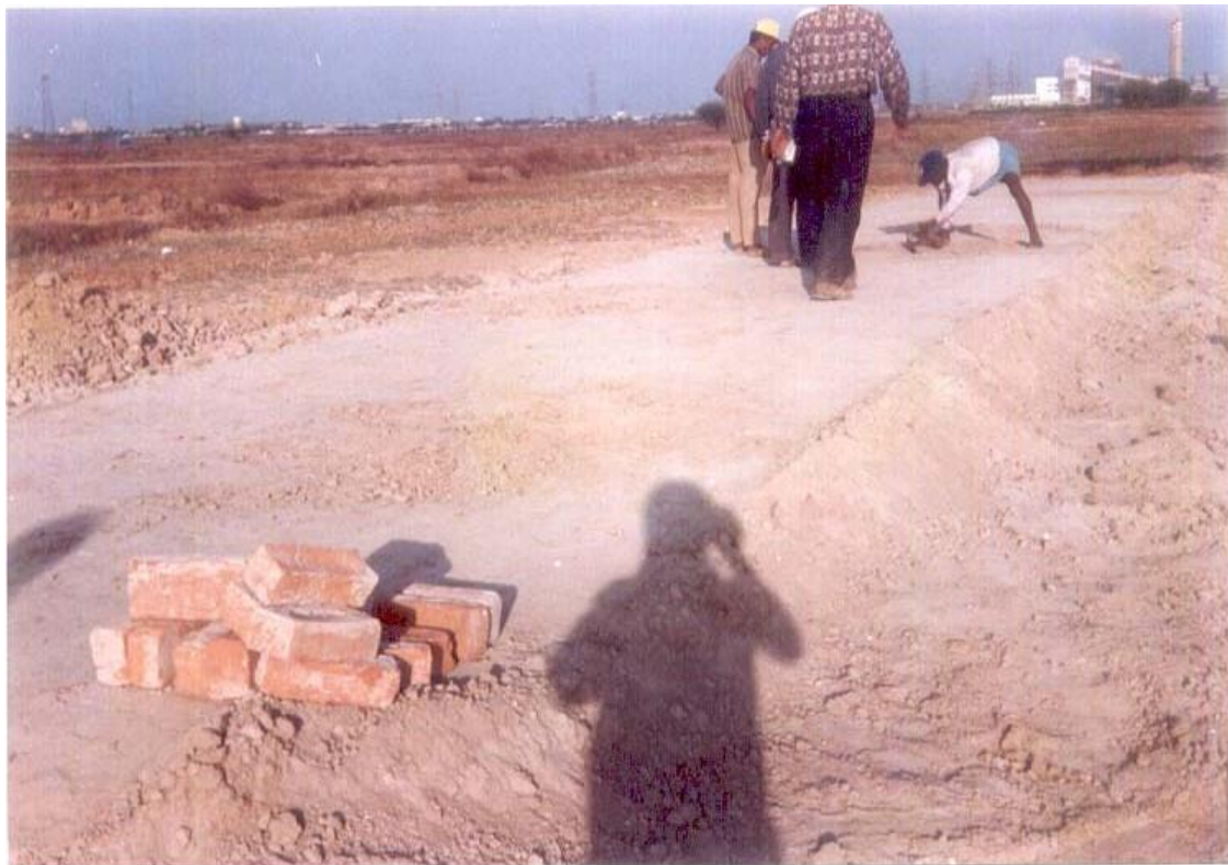
FIG.4 – VIEW OF COMPACTED SURFACE (SOIL WITH 20% FA)
